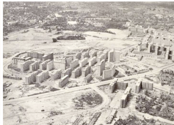
Figure 2. Construction of Toa Payoh, c. 1965. Image from Straits Times
