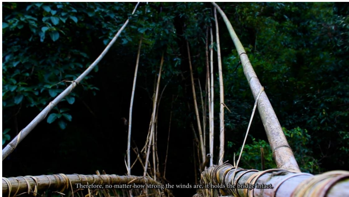
Suspensions to hold the deck of the bridge
