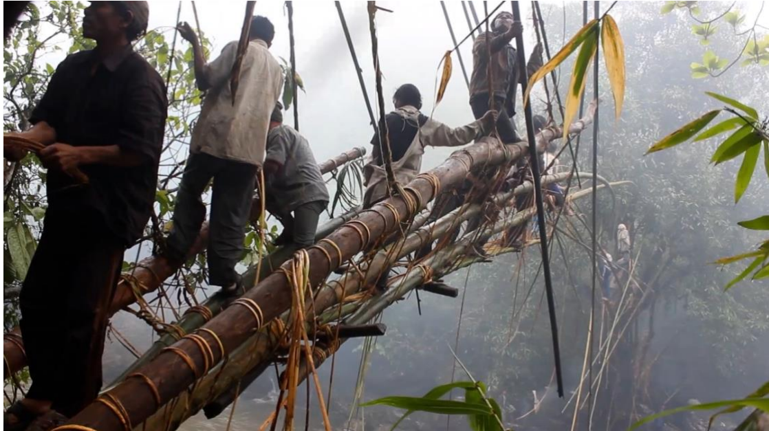
Construction of bamboo bridge
