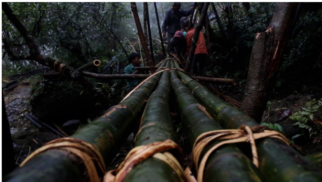
Deck of the bamboo bridge using bamboo ties
